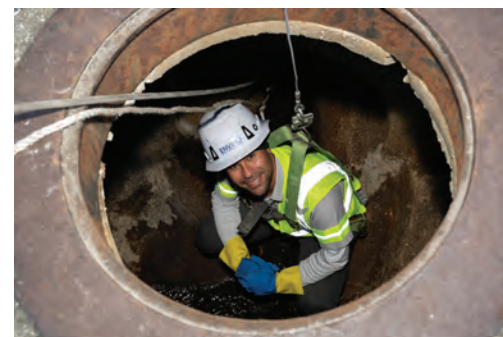
Edear Urreabarre enters a manhole for a visual inspection.
